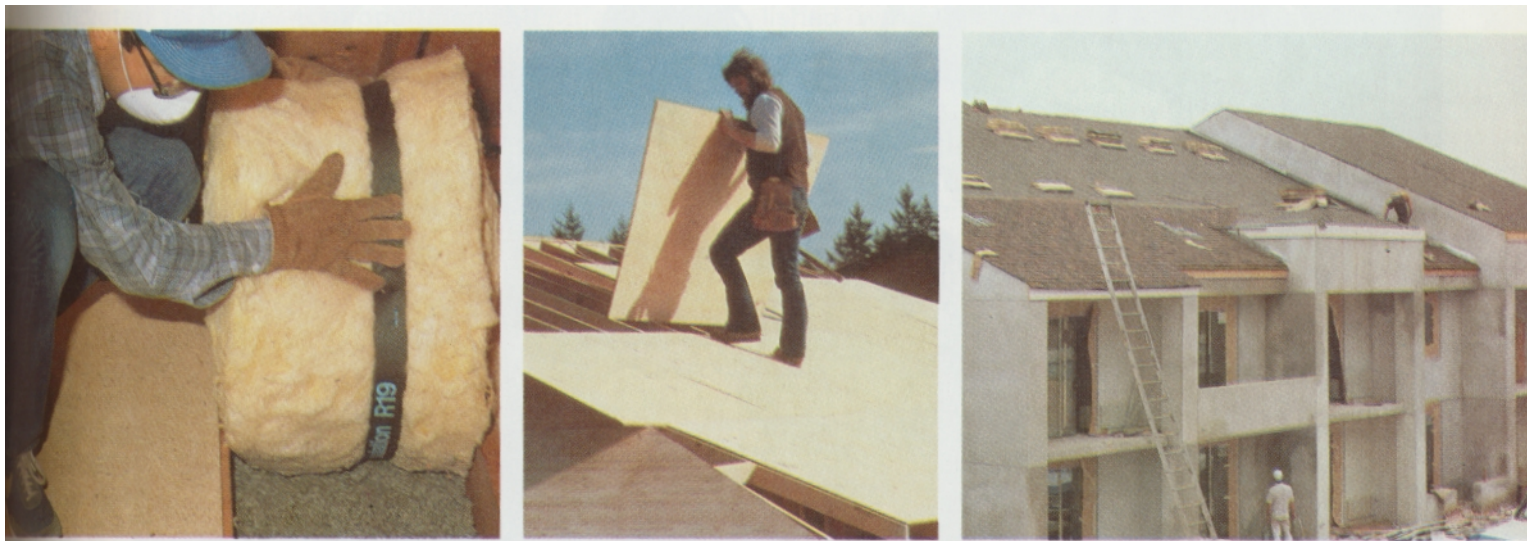
Safety tips for construction work. Left. When working with glass fibers, wear long sleeves, gloves, glasses, and a respirator. (Manville Building Materials Corp.) Center. Use extra care when handling large panels on windy days. Right. Ladders should extend above the roof edge at least 3 ft. See page 548. (Georgia-Pacific)
