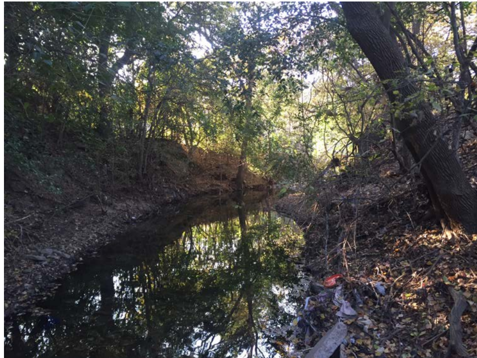
Above: A view looking west down Bouldin Creek as it runs south of the site. It appears heavy flow from upstream rain events has eroded the embankment beyond the traditional cross section of the creek. The erosion is currently undercutting the chain link perimeter fence.
